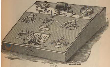
Brenner's Apparatus, including Stopper Rheostat, Galvanoscope, Faradic Coil, etc. (Galvano-Faradic Manufacturing Co.). This apparatus may be connected with any desired number of large cells in the cellar.
